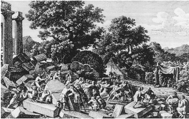
6. Work in progress: excavation of the temple at Bassae
